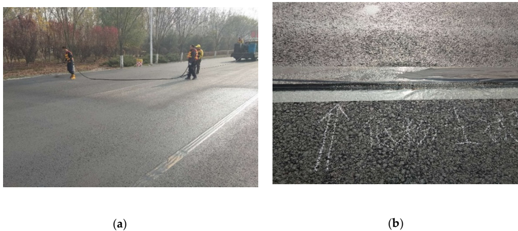
Figure 9. Spreading of functional Sand-fog seal: (a) Spraying; (b) Spray complete.
