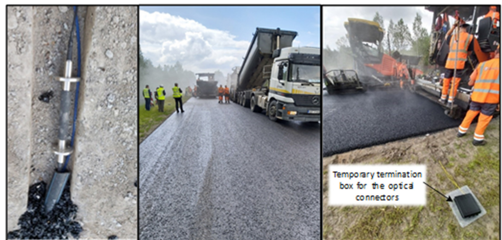
Figure 3. Photos from the construction process of road infrastructure where FBG sensors are integrated.
