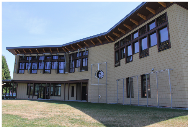
Figure 3 Monitored façades of the Annex building with Ornilux® glass at the Alaksen National Wildlife Area, Delta, British Columbia, Canada. Photo credit: K. De Groot.
