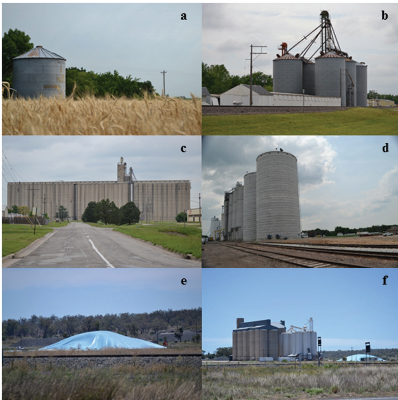
Figure 1. Grain-storage structures in Kansas (KS), United States, and Queensland (Qld), Australia. (a) A farm bin near Waterville, KS. (b) A country elevator in Rossville, KS. (c) A terminal elevator in Topeka, KS. (d) A rail-loading elevator in Hanover, KS. (e) A silo bag in Qld. (f) A concrete silo next to a depot near Toowoomba, Qld. Photographs: John F. Hernandez Nopsa.
