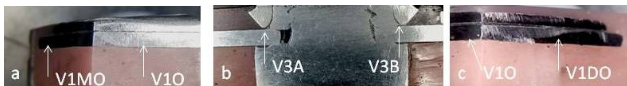
Figure 13. Sections through the framework assemble: (a) V1MO, V1O; (b) V3A, V3B; (c) V1O, V1DO.
