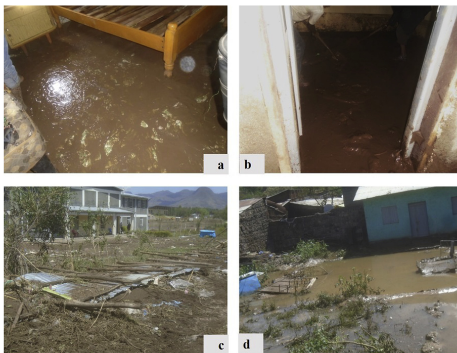
Figure 5. Households (a,b,d) and fences (c) affected by flooding and clearing the mud sediments (a,b).
