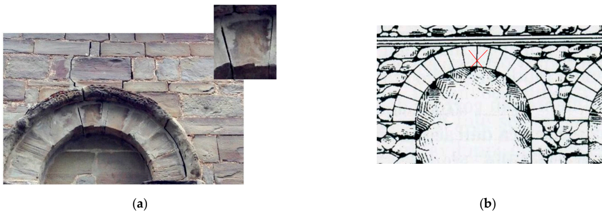
Figure 18. (a) Shear loads and differential subsidence can cause ring stones to slide on another, (b) Titanium rods, inserted in holes drilled in adjacent blocks, could be used to prevent sliding.
