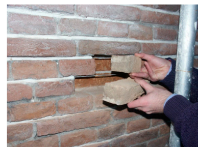
Figure 16. Shear reinforcement of wall panels: the tensile strength of historic masonry is typically very low. Under the action of an earthquake, shear cracking is a common failure mode. Metal rods can be embedded into the mortar joint to absorb tensile stresses under seismic loading. Rods are hidden from view, and this can be important when the fair face aspect of the masonry needs to be preserved.
