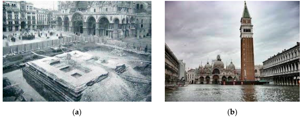
Figure 8. (a) Reconstruction of the St. Mark bell tower, Venice, Italy, in the 1910s, made of bricks and stones over timber piles; (b) the bell tower, after reconstruction, with the flooded square and foundations. High tide often causes flooding in St. Mark square.
