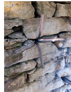
Figure 15. Examples of leaf-to-leaf connections; connections in historic masonry constructions are an area of concern. Metal ties can be inserted using lime mortar.
