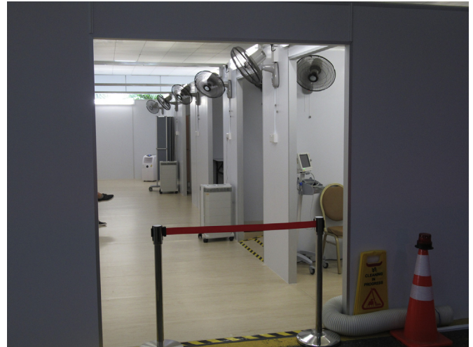
Figure 2 Naturally ventilated triage area installed in a converted car park adjacent to the emergency department.
