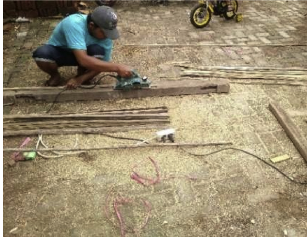
Fig. 6. Exfoliating the inside of the bamboo and adjusting the dimensions of the bamboo to the reinforcement plan.
