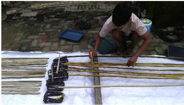
Fig. 9. The initial surfacing of Sikadur®-752 adhesive.
