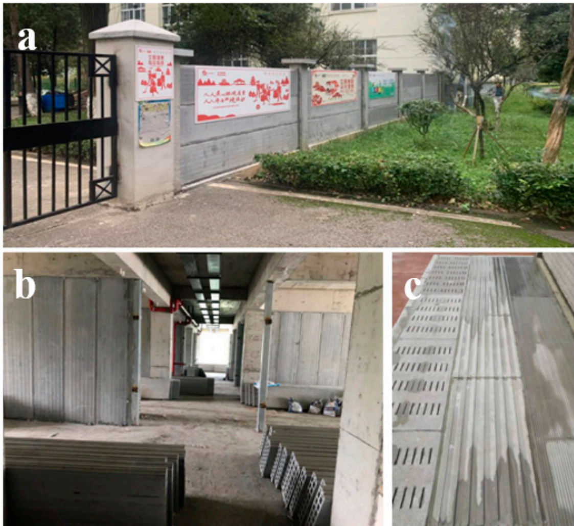
Figure 10. (a) PG exterior wall in the campus of Guizhou Institute of Technology produced from HPG-E composites; (b) PG interior wall panel produced from HPG-E composites; (c) PG pavement produced from HPG-E composites.
