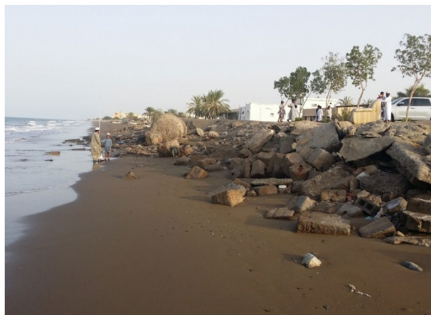
Figure 2. Construction debris used to break the sea waves in the study area.
