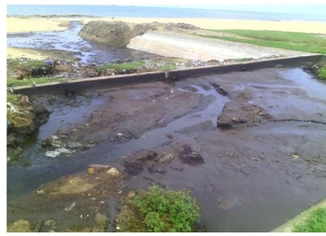
(e) Maturation basins and discharge of the effluent by natural outlet
