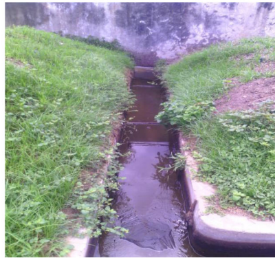
(c) Wastewater discharge channel to the basins
