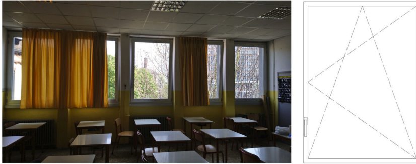
Fig. 6. Shape and typology of the windows found in classroom C3D. Type C: Tilt-and-turn windows with one casement.
