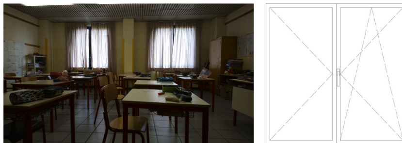
Fig. 4. Shape and typology of the windows found in classroom A1C. Type A: tilt-and-turn windows with two casements.
