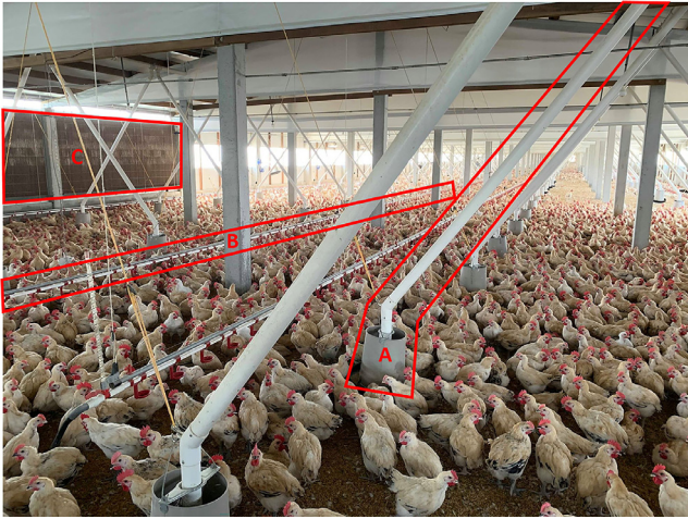
Figure 1. Configuration of the chicken farm: (A) feeding pipeline, (B) nipple drinkers, and (C) cooling pad system.
