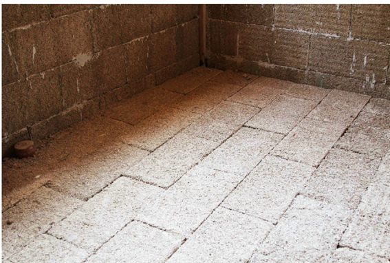
Figure 6. Hempcrete in floor covering [193].
