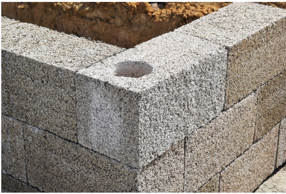
Figure 4. Hempcrete blocks in construction [193].
