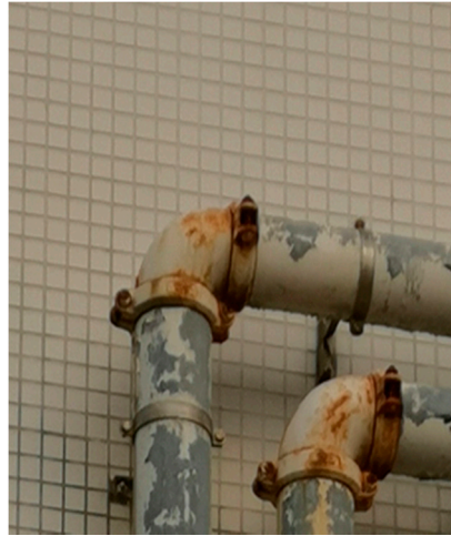
Figure 8. Mounting brackets near two elbow joints found in Yuen Long, Hong Kong, China.
