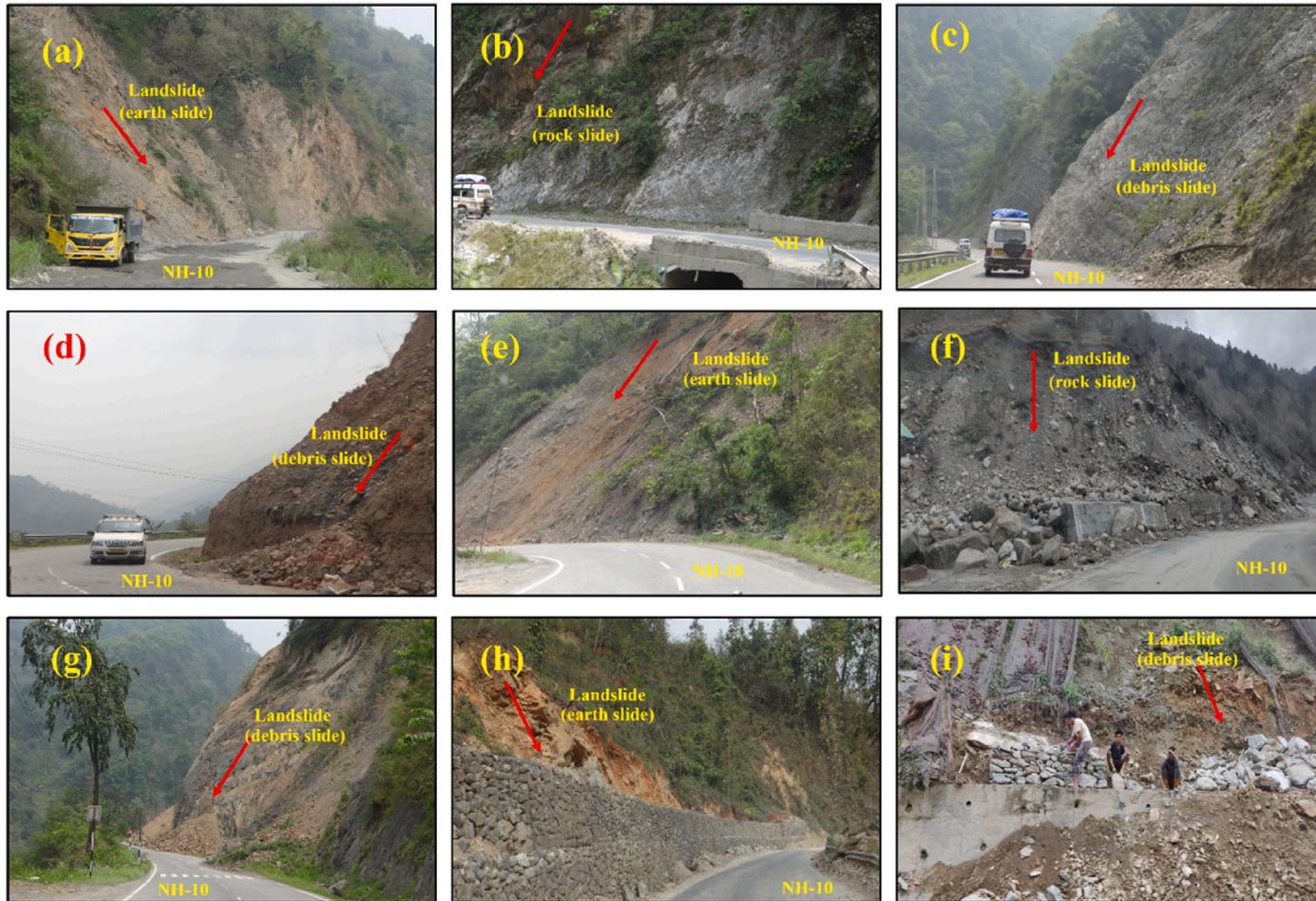
Fig. 2. Field photographs of landslides within the study area: (a), (b), (c), (d), (e), (f), (g) Different landslides occurring places along NH-10 in Upper Tista Basin; (h), (i) Protection against landslide.
