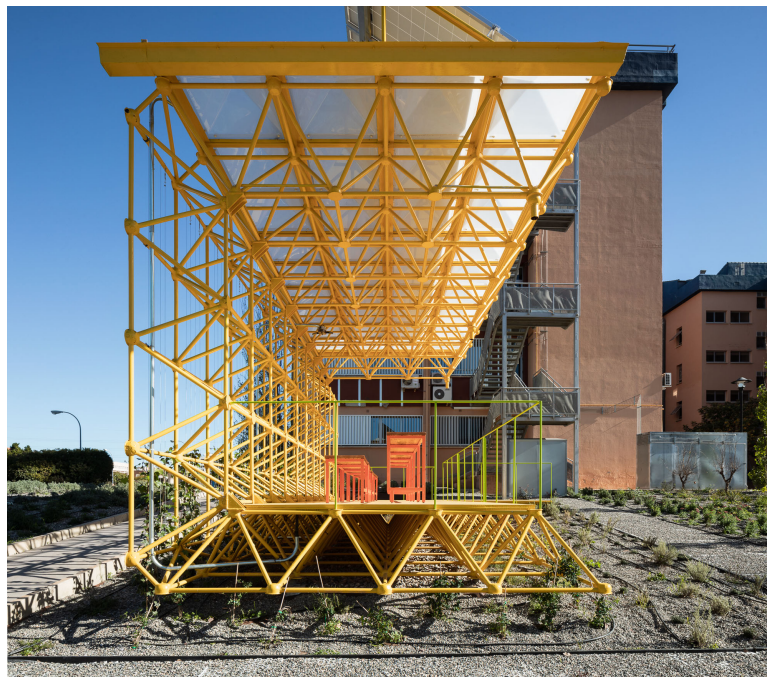
Figure 3. Structural order of the Smart Tree architecture.
