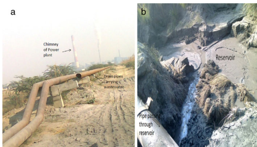
Figure 2 a) Harduaganj Thermal Power Plant draining wastewater into the reservoir b) Present Scenario: Degraded condition of reservoir.
