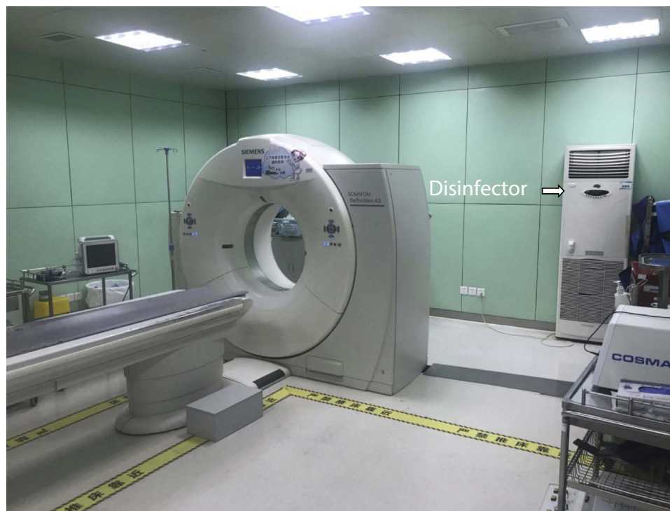
Figure 1 CT operation room for interventional procedures with sterilization of the room.
