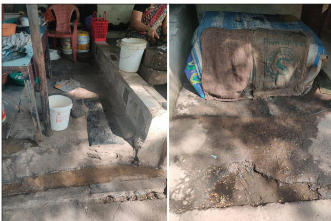
Figure 3: Improper water disposal and open drain
