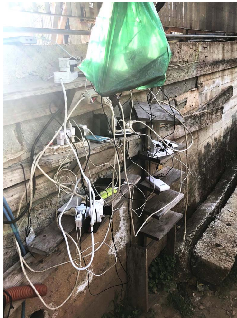
Figure 4. An electrical hub in a shack in the San Ferdinando settlement where residents charge their mobile phones.
