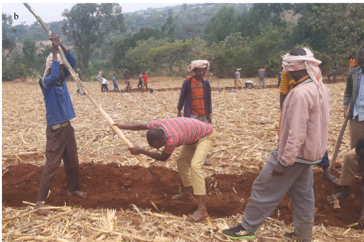
Fig. 2. Soil bund constructed through community participation (a) design of the soil bund (adopted from Refs. [31,33]) and (b) participation of farmers in constructing soil bund (Photo documented by Omo Nada district's agriculture and natural resource office).
