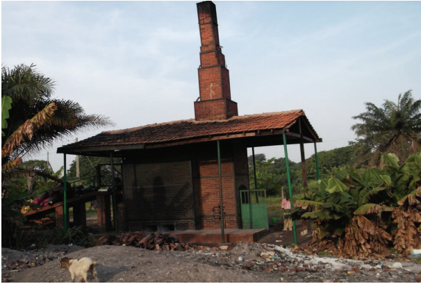
FIGURE 1: Showing the incinerator and the ash dumping point.
