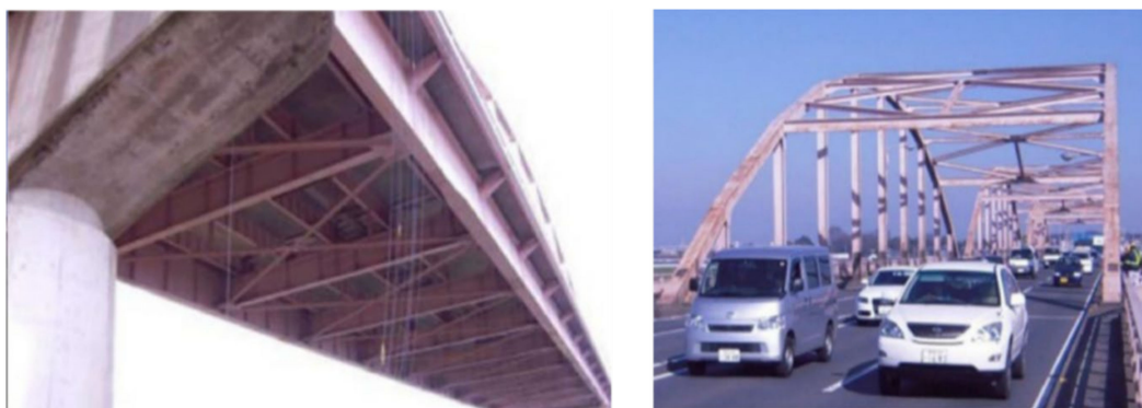
Figure 18. Two views of a steel arch bridge [173].
