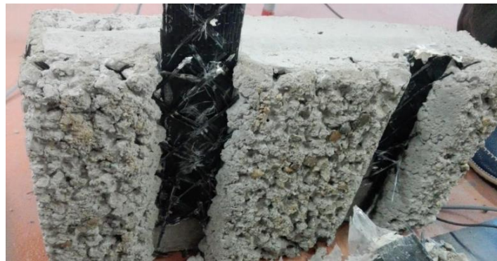
Figure 5. Failure mode of A-IM cases combining mesh debonding from the CFRP sheet and mesh breakage.
