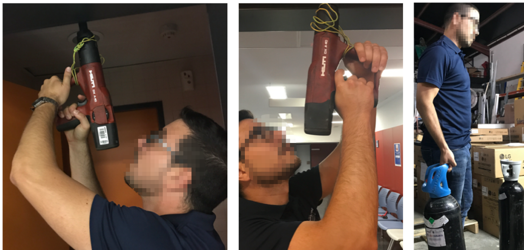
Figure 1. Examples of industrial maintenance tasks: work tasks with the hands overhead in drilling holes into the ceiling and lifting and carrying loads. All the participants that appear in the figure have provided written and informed consent for its publication.
