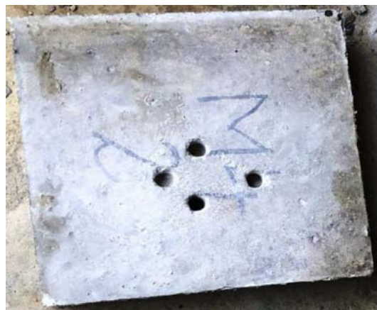
Fig. 4. Drilled holes of 10–20 mm and 25–35 mm depth for obtaining samples for chloride ion penetration test.
