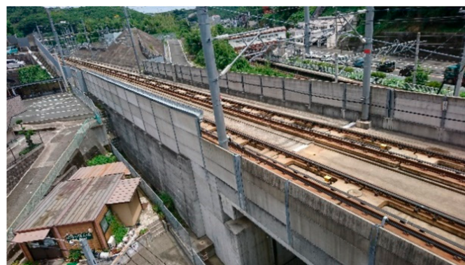
Figure 4. Shinkansen railway line. The forward barrier is 2 m high and the back barrier is 3 m high on the left-hand side.
