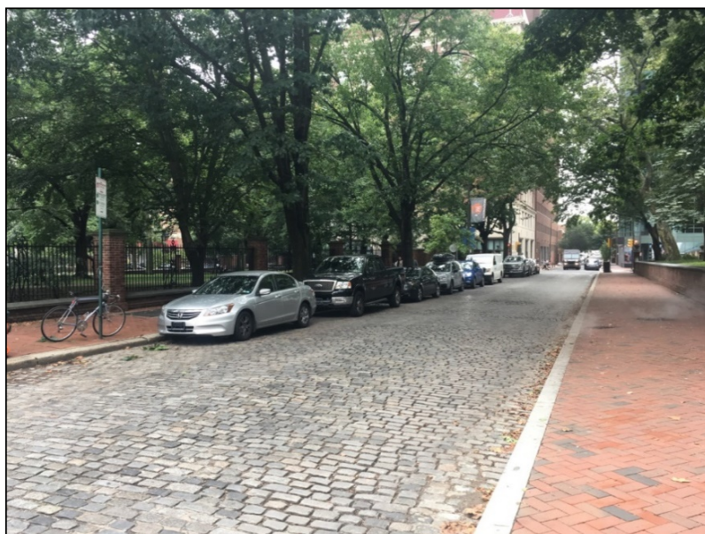
Figure 2. A Philadelphia street paved with granite block historic paving material, located at 102 S. Independence Mall E.
