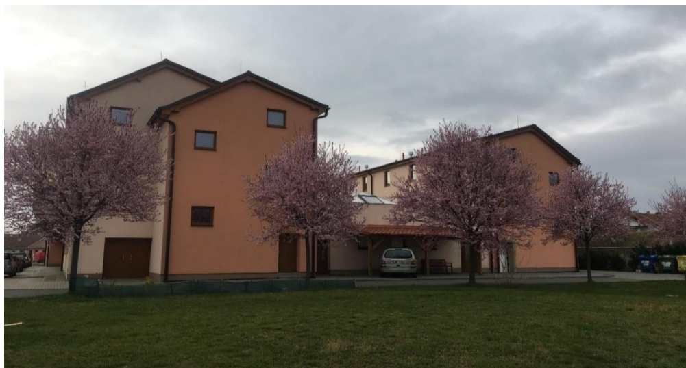
Figure 5. A view of the social care home for elderly people from the courtyard in Vranovice. Source: K. Charvátová (2021).
