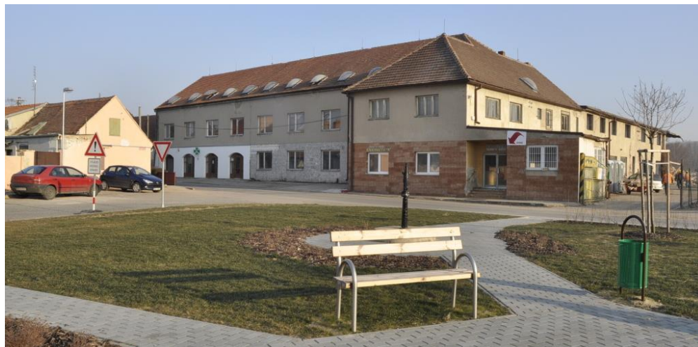
Figure 1. A view of the administrative building of the former socialist agricultural cooperative in Vranovice. Source: [58].
