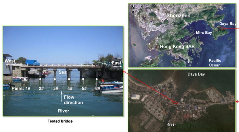
Figure 1. Geographic location of The tested bridge.
