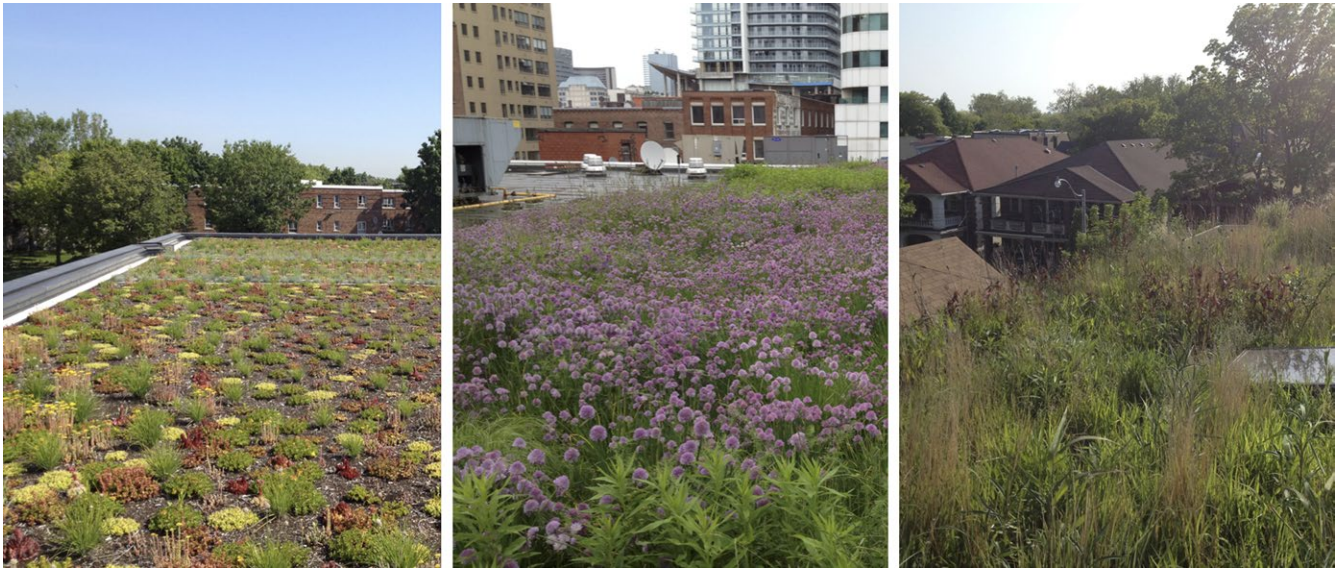
FIGURE 1 Three extensive green roofs all from Toronto, Canada (from left to right): Regent Park swimming pool, Mountain Equipment Co-op, a residential home
