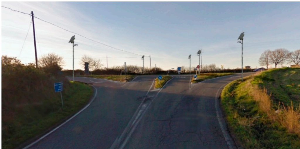
Figure 6. Test system in the field.
