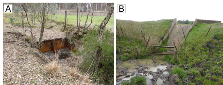
Fig 3. Erosion control structures, constructed in the late 1960s and early 1970s, in small headwater streams in the Bryan Creek catchment. (A) 'Drop structures'—small grade control structures which span the channel and trap sediment, (B) concrete chutes which slow erosion by preventing nickpoints from migrating upstream. Photos courtesy of Glenelg Hopkins Catchment Management Authority.
