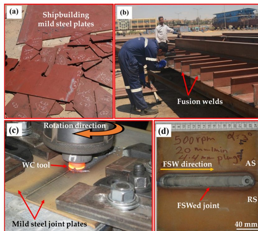
Figure 1. (a,b) Images of mild steel shipbuilding plates and conventional fusion welding during the manufacturing process, respectively. (c,d) Images of the FSW process of mild steel plates and a top view of the produced butt joint, respectively.
