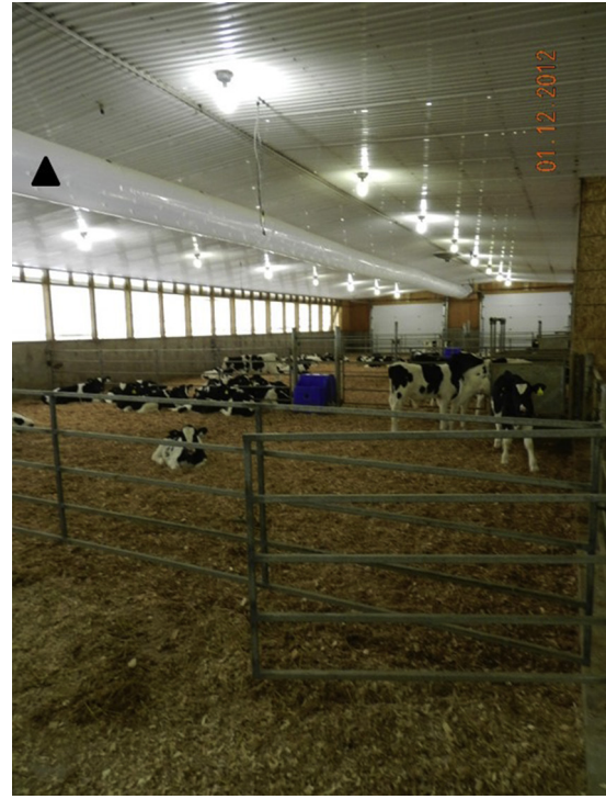
• Fig. 4.63 Indoor group housing with supplemental air provided through positive-pressure ventilation. The black triangle indicates the positive-pressure tube.
