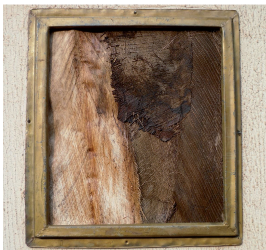
Figure 4. Natural net (from axiles of cocoa-nut tree) hoisted with welded S/O channel/grip device on a window. Note that each piece has a different hole size.
