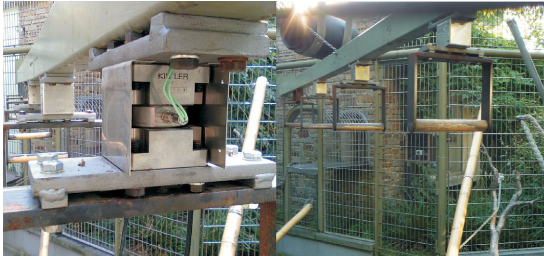
Fig. 2. Detail of Kistler force transducer installed in setup 2.
