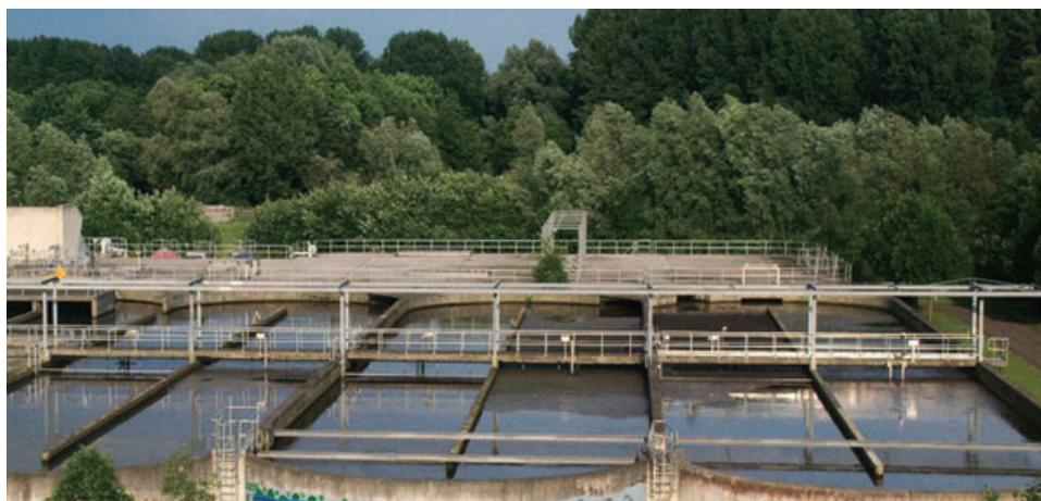
Fig. 1. Wastewater treatment plant near Arnhem, the Netherlands (photo M. Galardini).
