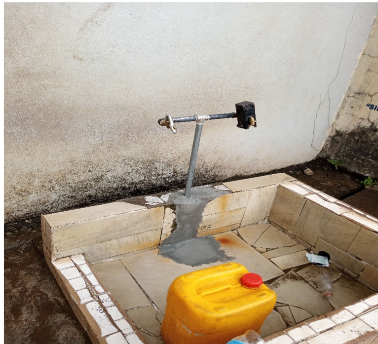
Figure 6. A typical example of one of the standpipes in Brookfields connected to the pipe network. The tap is closed after use by the people.
