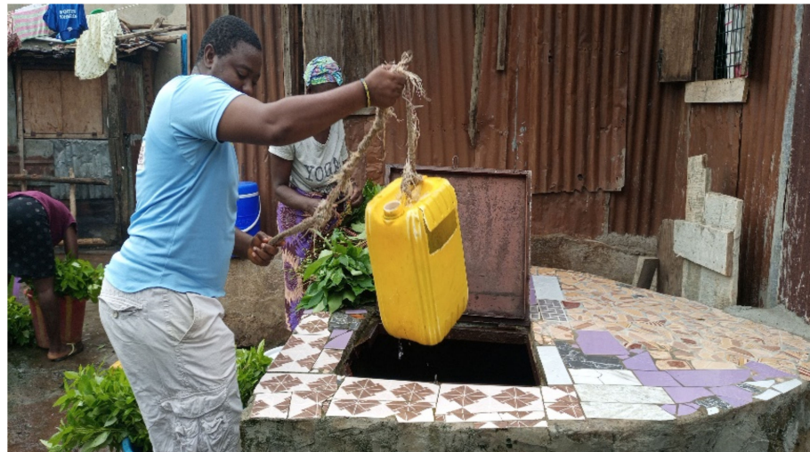
Figure 4. Sources of contamination at a well. Leafy vegetables are washed on top of the well, and that same water may drain back into the well. While the woman washes the vegetables, the man fetches water using a plastic container hung from a rope. The lid or cover is also prone to corrosion as it is made of iron and can be another potential source of contamination.
