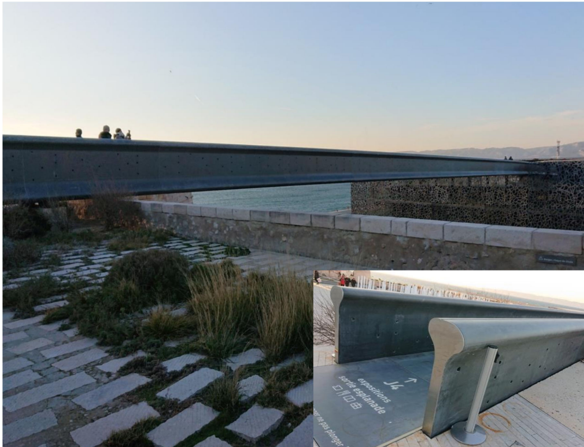
Figure 1. Application of ultrahigh performance concrete (UHPC) in MuCEM pedestrian bridge (Marseille, France).
