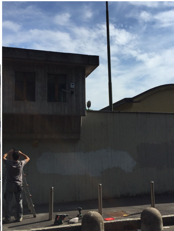
(b) Sensor placement in the facade
