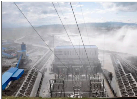
Figure 7. Prototype observation of powerhouse rainfall.
