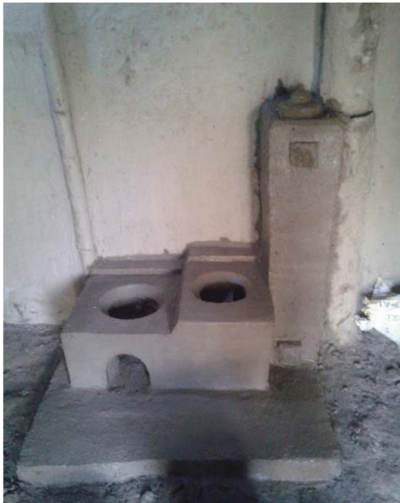
Figure 4 Locally constructed, improved cookstove installed in Nepal.
