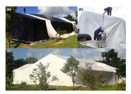
**Figure 1** (a) Inner ethylene vinyl alcohol tarp (black) with skirt around the building perimeter; (b) clamping seams of the outer vinyl tarp; (c) fully tarped building.
