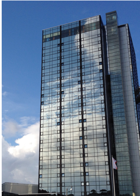
Figure 1 Sky reflected in the windows of a high-rise building in central Gothenburg, Sweden. Photo by Anders Ödeen.
