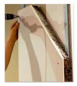
Figure 2. ICB glued to gypsum plasterboard in an Internal TICS (ITICS) [10].
