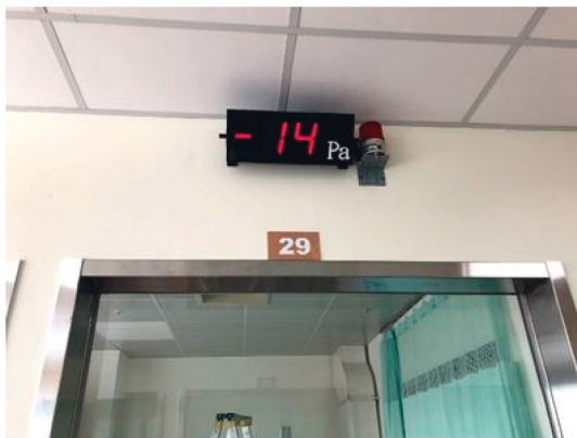
FIGURE 16: Negative pressure at the experiment site.
