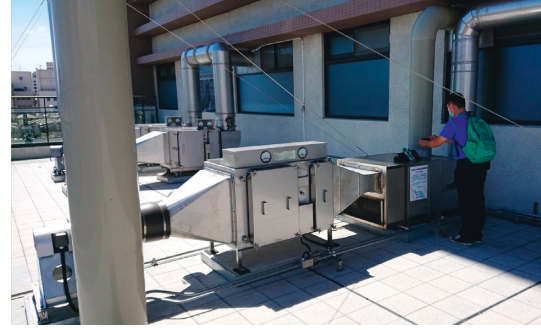
FIGURE 12: Picture of the completed full-outer-air-intake natural air-conditioning system for negative pressure isolation wards.
