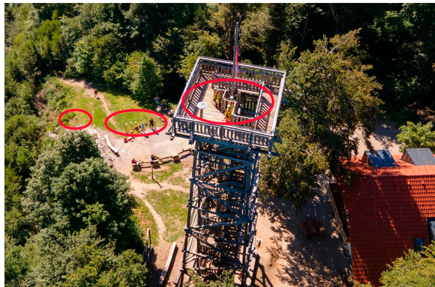
Figure 3. Vertical profile of jamming at the Stara Vrhnika location, top–down view, acquired by a Mavic Air 2, DJI drone. The upper metallic fence structure and flagpole are grounded.
